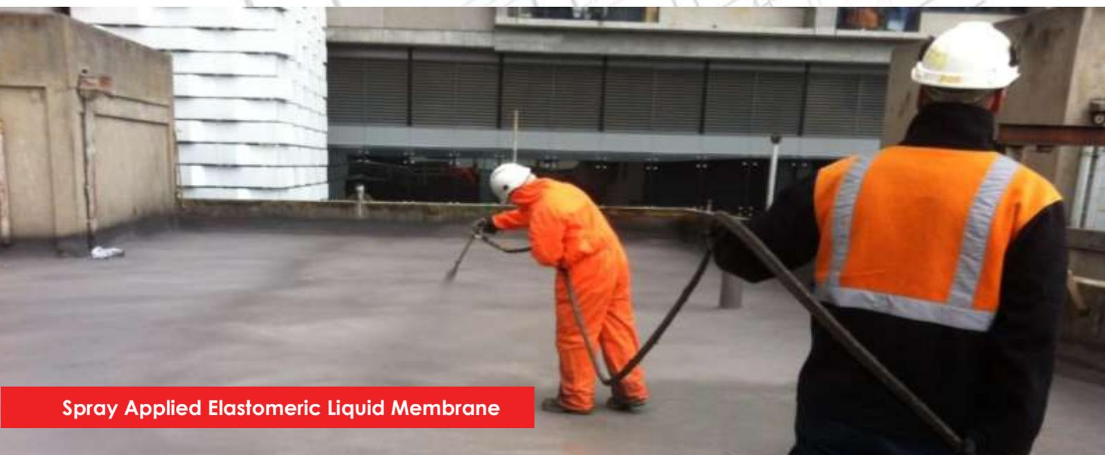
Spray Applied Elastomeric Liquid Membrane
